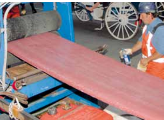
On-site impregnation of NORDIPIPE™ (2)
