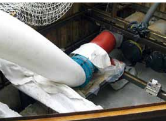
Installation of NORDIPIPE™ liner
