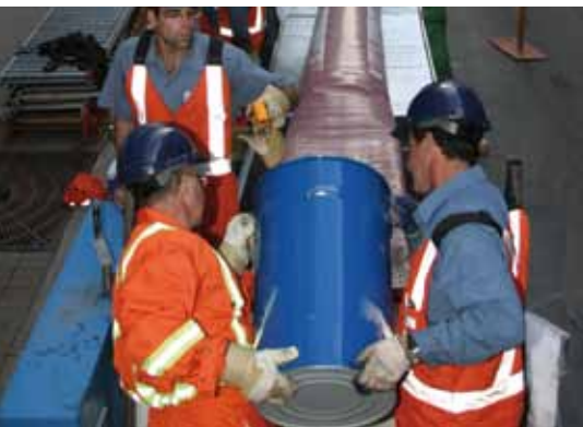
On-site impregnation of NORDIPIPE™ (1)
