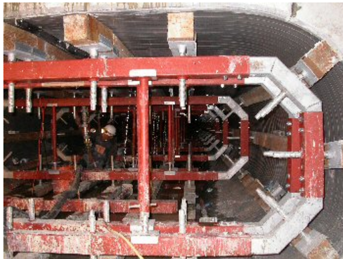
Figure 5. Installed Bracing
