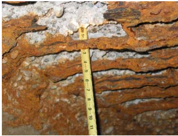
Figure 2. Soffit Corrosion
