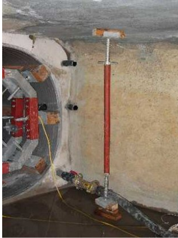
Figure 6. Grout injection behind the braced liner
