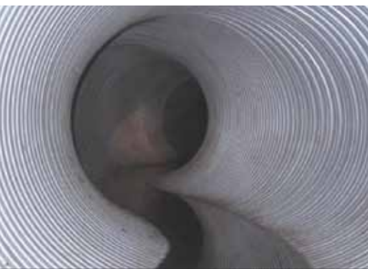
Rehabilitation of bends
