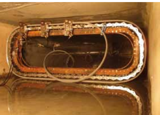
Rehabilitation of custom shape
