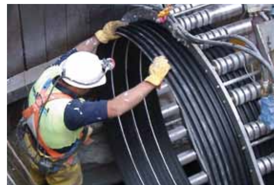
SPR™ PE liner being produced by the winding machine
